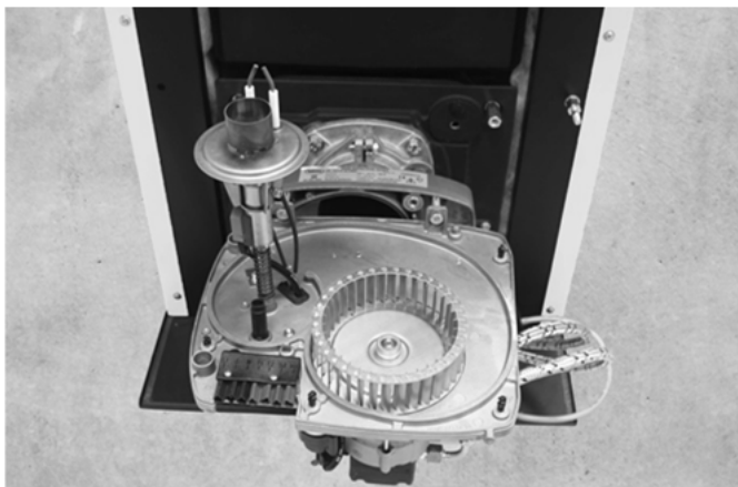
Abb. 36: Brenner in Serviceposition
