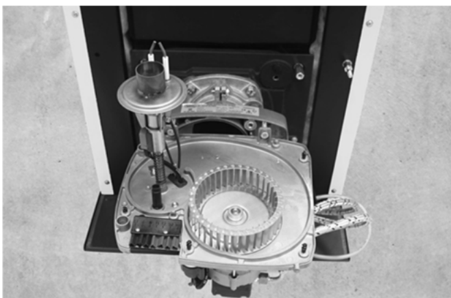
Abb. 36: Brenner in Serviceposition
